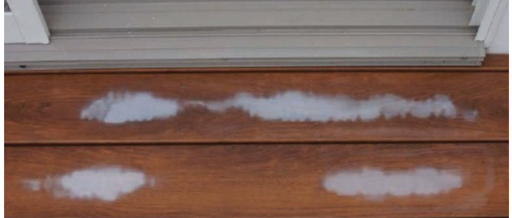
Example of discoloration that can be caused by using these products on Zuri Deck.
